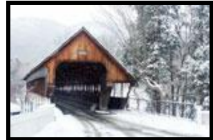
Covered bridge Woodstock
